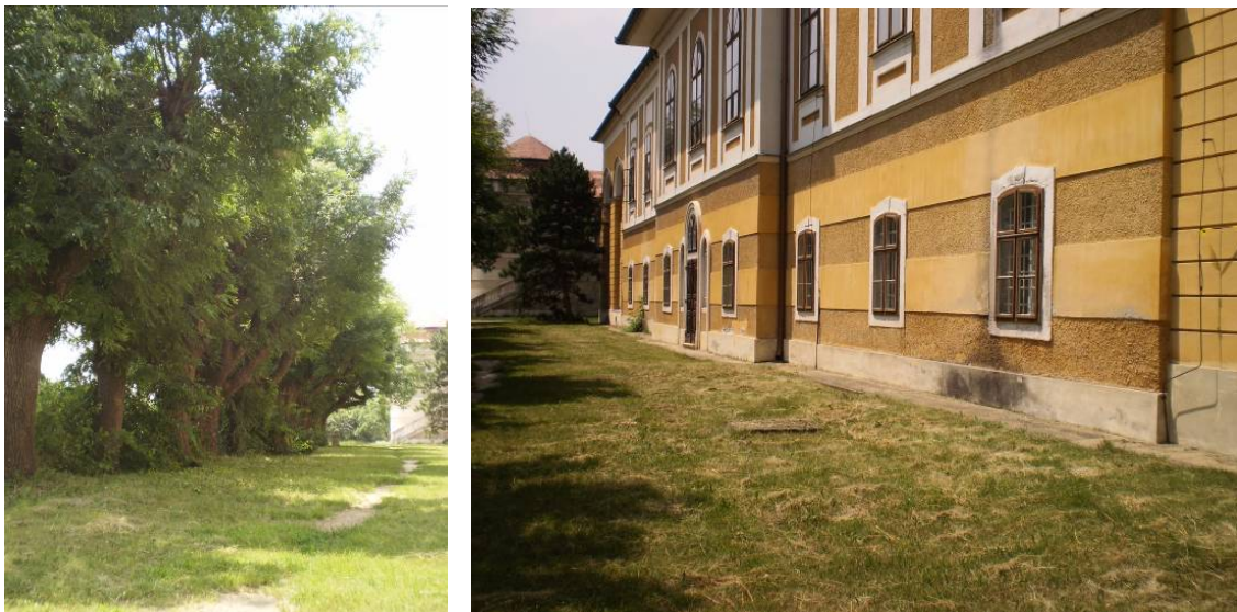
Figures 7& 8. Views from the backdoor of the main building on the 1 st terrace. (photos taken by Annika Pöyhtäri).
