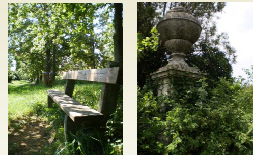
Furniture & Structures - Some old stone columns, vases and other structures still remain - Old benches in a poor shape
