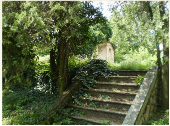
Ivy has taken over many structures on the site
