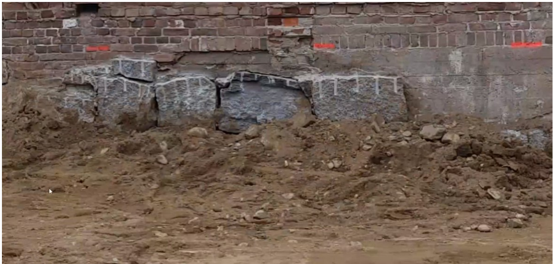
Figure 17: Loose stone foundation (left) and RC beam foundation
