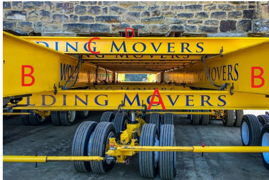
Figure 1: Steel support frame on dollies (Wolfe House & Building Movers, 2016)
