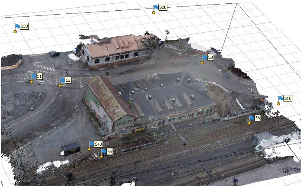
FIGURE 19. Point cloud exterior
