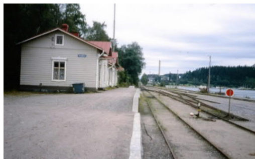
PICTURE 15. Vesijärvi railway station and railway yard in the early 1990s. (Lahden Kaupunkiympäristö 2020)
