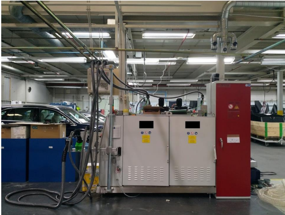
Picture 8 Filling machine in the middle of installation.
