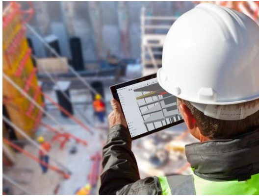
Figure 17 Trimble Connect use on site.(Trimble MEP, 2020)
