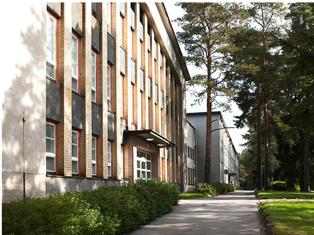
Figure 8. Vaasa factory and office building. Picture from Vaasa Factory presentation 1997 (ABB internal network)
