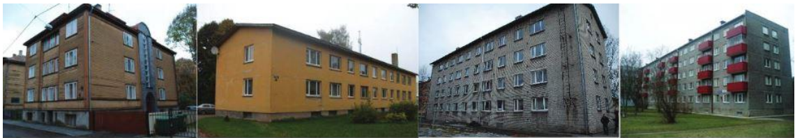
Figure 7. Typical Soviet-era buildings in Estonia. From left to right: wooden, large block, brick, large panel
