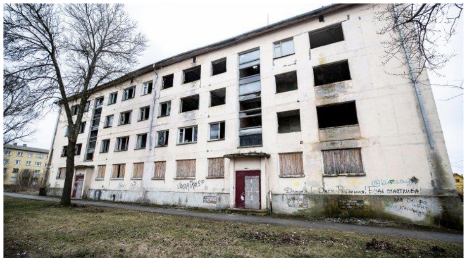
Figure 4. Abandoned Hrustseva in Kohtla- Järve
