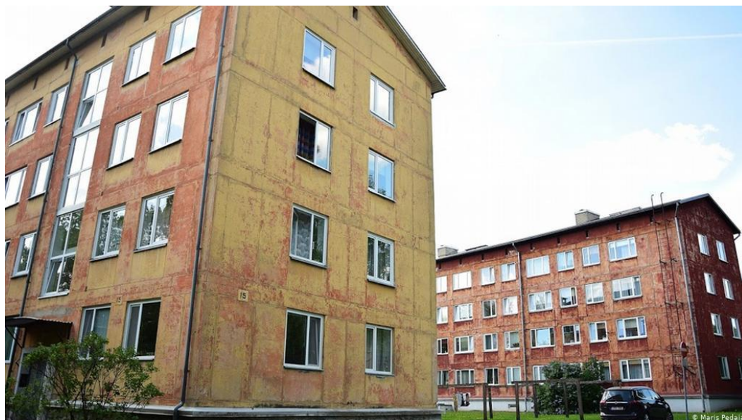
Figure 12. Hrustsevka before renovation [4.]
