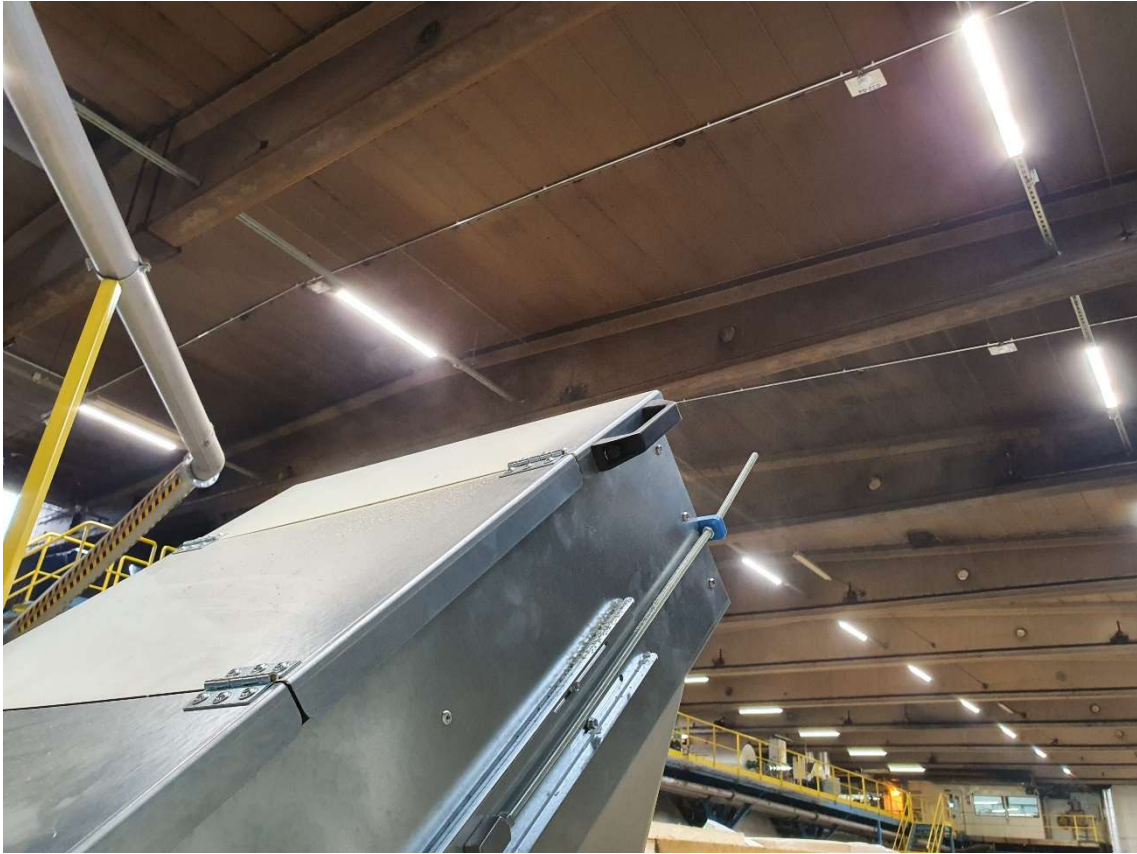
Figure 33 Dust emissions from the conveyor housing (Kohvakka, 2020)
