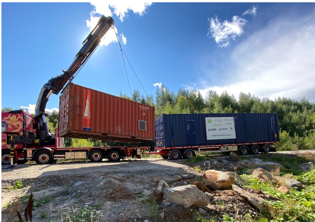
Figure 6. Morecovery containers being set up at the Hitura mine site (source: Pesonen 2020).
