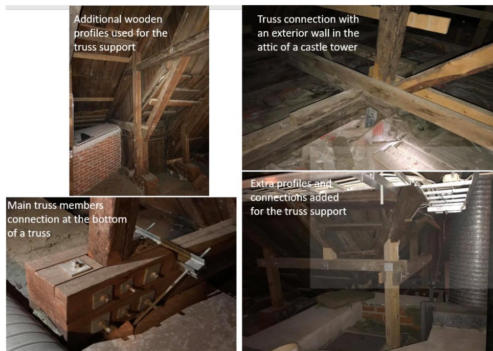
Figure 33. Truss connection and irregular timber profiles in the main castle attic
