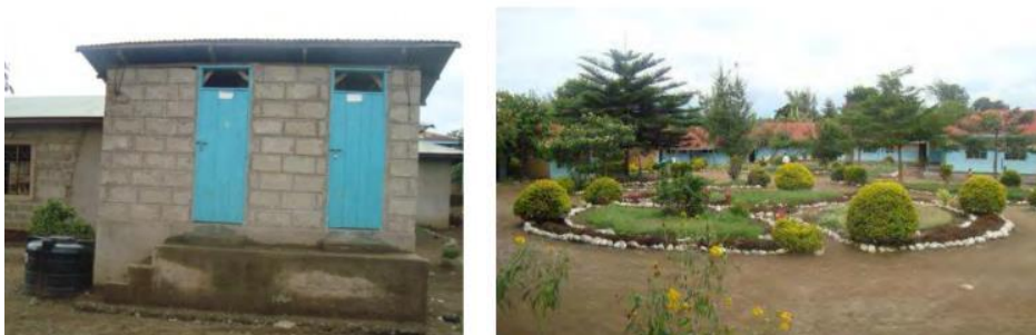
PICTURE 26. Urine diversion dry toilets in a school compound, built by the ROSA project in Arusha. (Senzia 2011)
