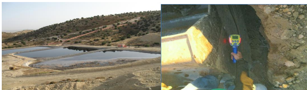
Full Leachate basins need treatment and to be powered by future energy & Biogas detection tests at the old site at Bikarane in Agadir
