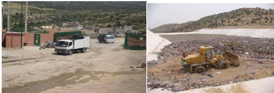
New landfill at Tamlast in Agadir
