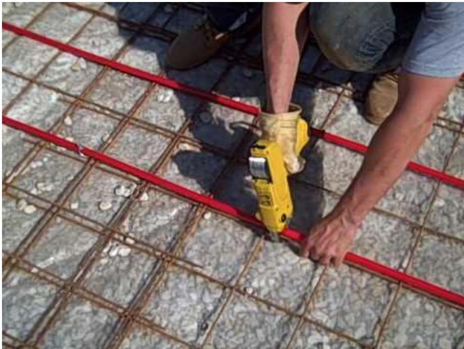
PICTURE 2. Heating pipes secured with a rebar tier (Max USA Corp 2011)
