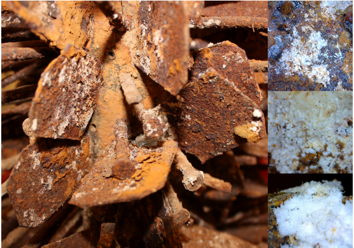
Picture 13. Corrosion, dirt and calcium carbonate deposits. Photos on the right are taken with a microscope camera (magnification 50 and 200).
