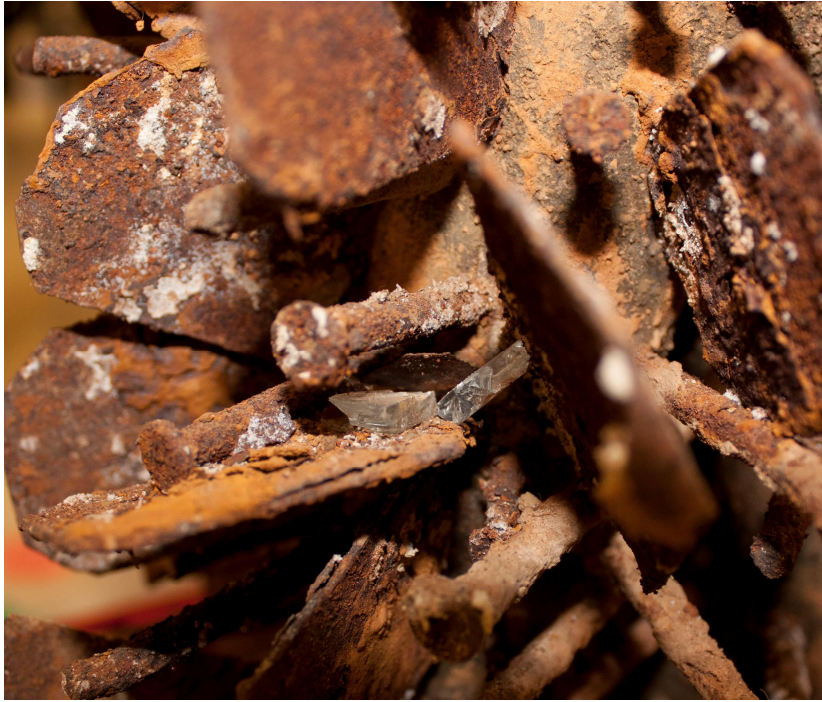
Picture 17. Corrosion and debris on the surface of the object.
