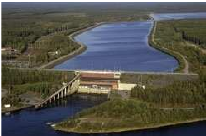
FIGURE 9. Hydro power plant in Iijoki in the north of Finland (Pohjolan Voima Oy).
