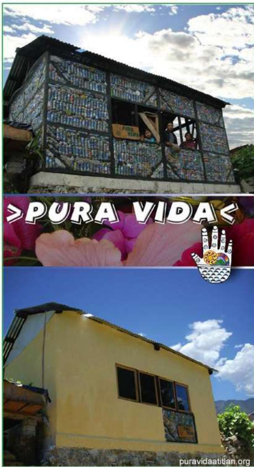
Pic 19 Eco-Bricks used in building.
