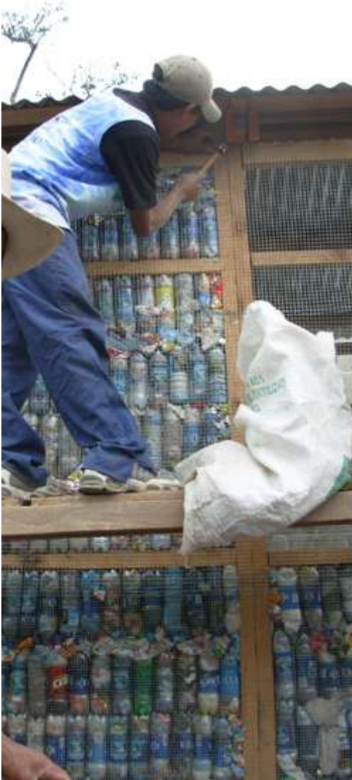
Pic 18 Construction of Pura Vida eco brick wall.
