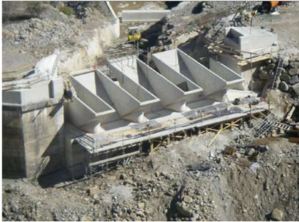
Figure 6. Photo of a PK Weir of Gloriettes dam in France (Schleiss, 2011)
