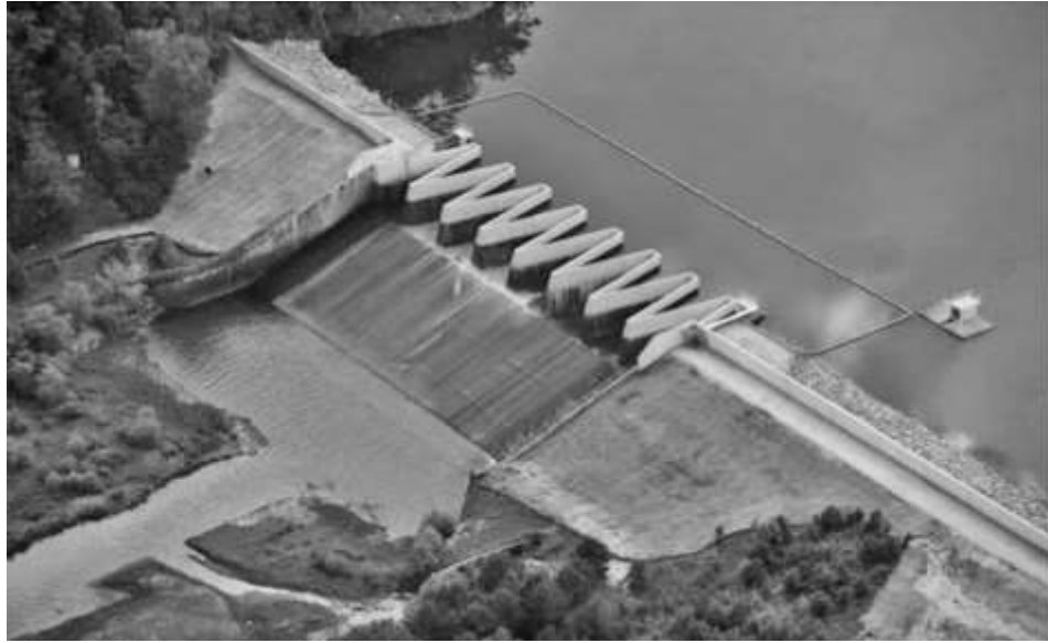
Figure 5. Photo of the Trapezoidal Labyrinth Weir in Lake Townsend dam, Greensboro, North Carolina, USA (Schnabel Engineering, 2020)
