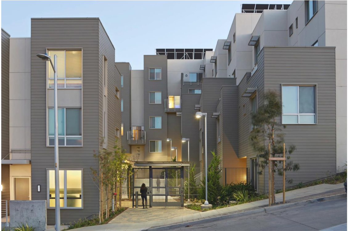
Kuva 18. Näkymä sisäpihalle. ( https://www.archdaily.com/870040/hunters-view-housing-blocks-5-and-6-paulett-taggart-architects/59002dbae58ece9ed7000182-hunters-view-housing-blocks-5-and-6-paulett-taggart-architects-photo )
