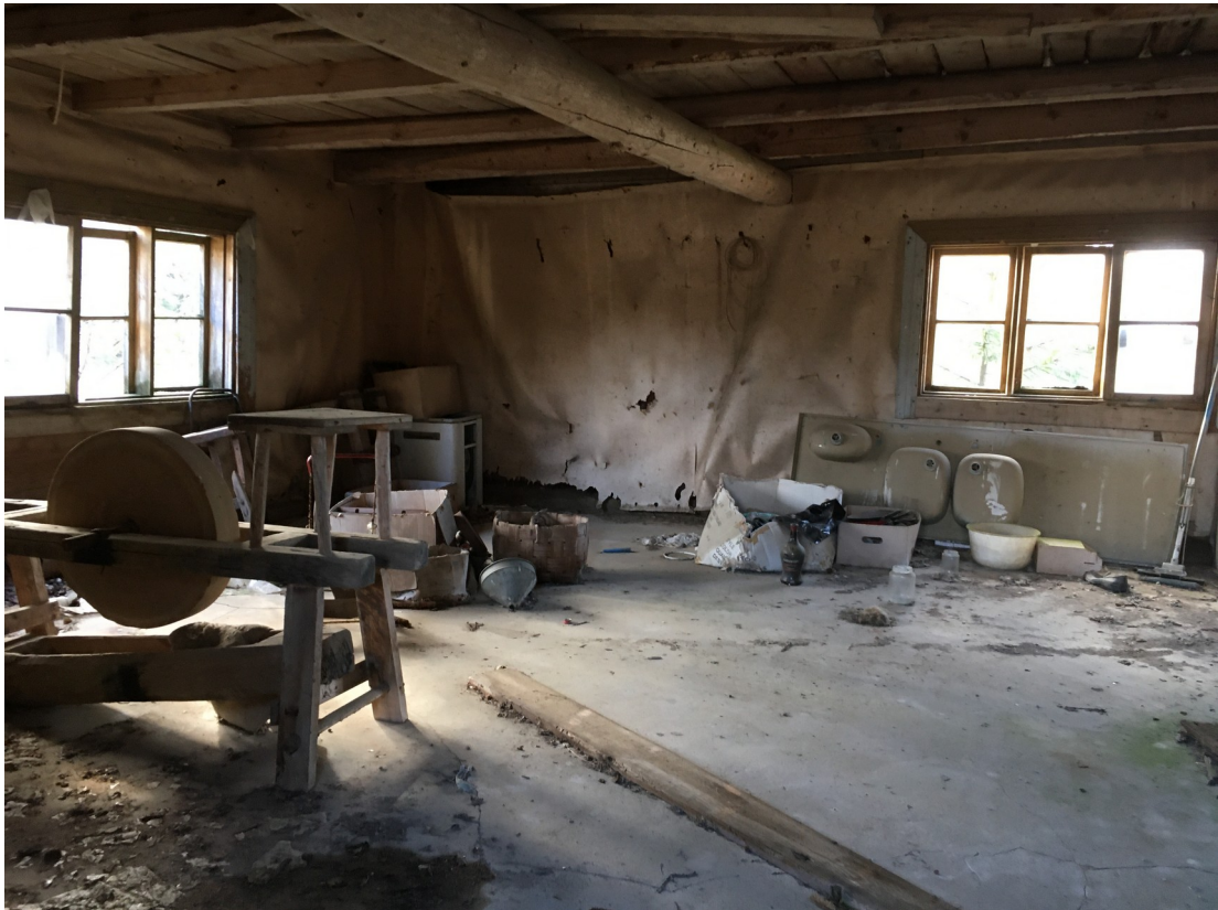
PICTURE 4. Interior of an abandoned house in Pirkanmaa, Finland. (Vesiväki 2020)
