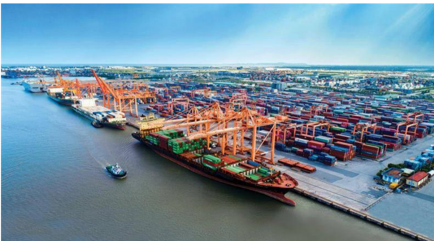
FIGURE 2: Hai Phong port (Ministry of Transport 2019)
