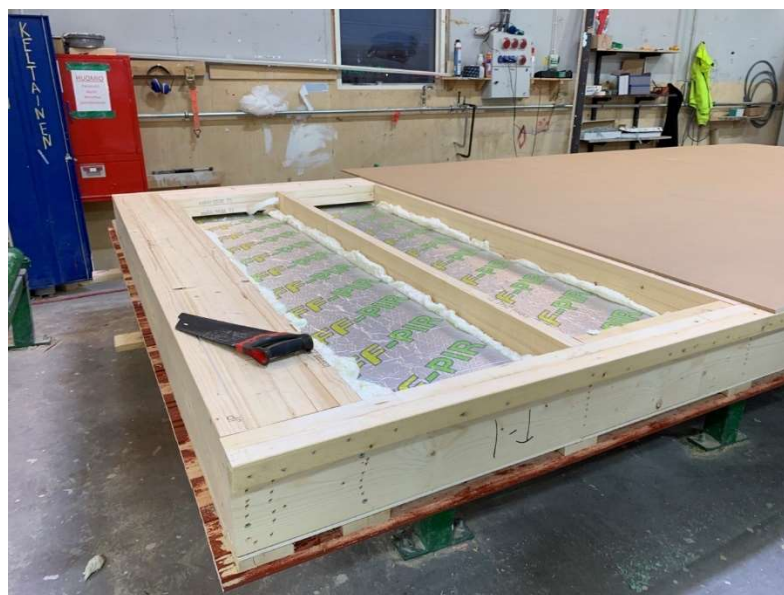
Figure 4.6. The long wall on the assembling table
