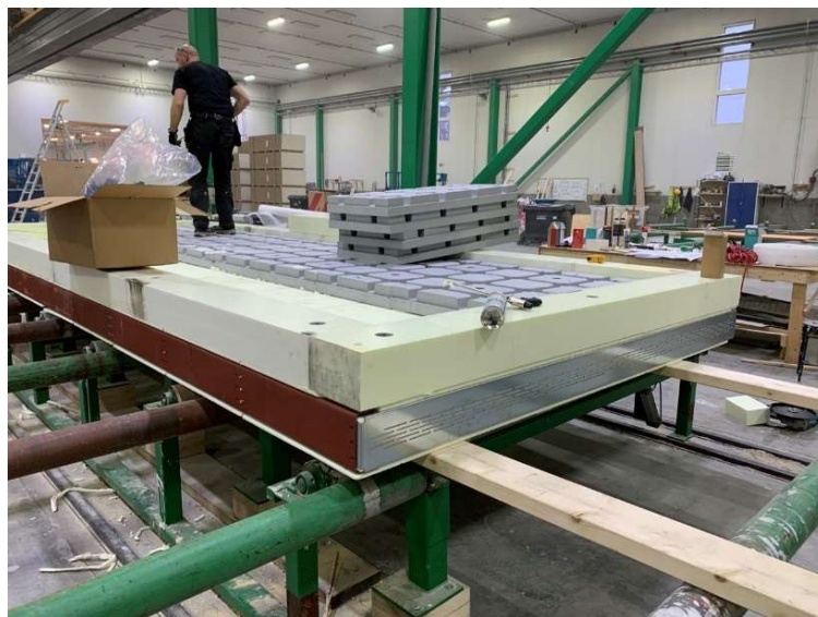
Figure 4.9. The floor structure on the assembling line
