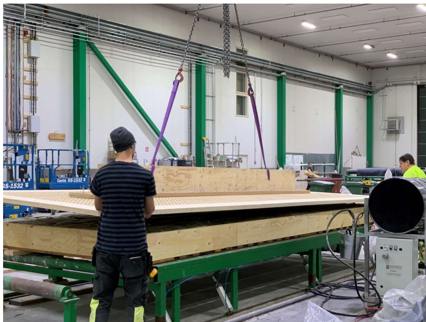
Figure 5.6. Process of glueing LVL-plate to the frame
