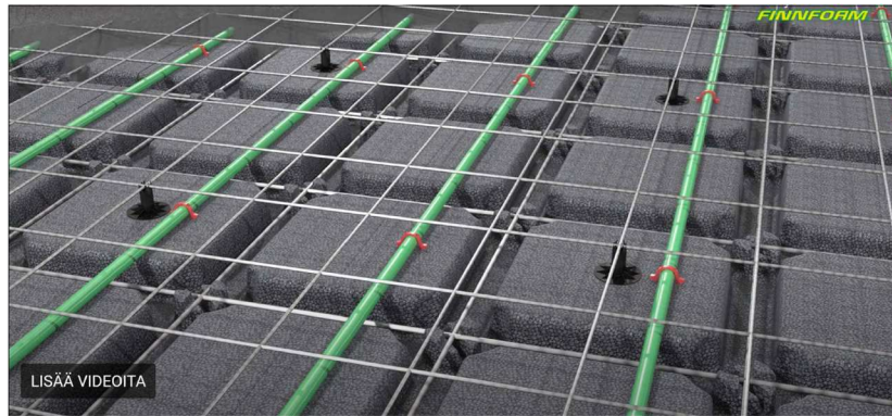
Figure 4.10. Prepared structure for concrete pouring (picture: FinnFoam)
