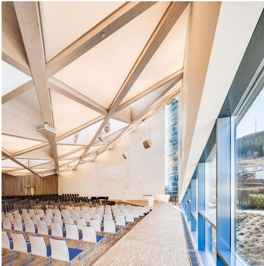
Figure 2.1. Glulam roof structure in Algard Church (photo: archdaily)
