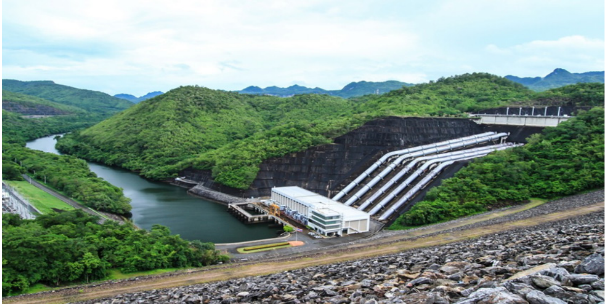
FIGURE 24. A pumped hydro storage power plant in Thailand (Shutterstock, 2021).
