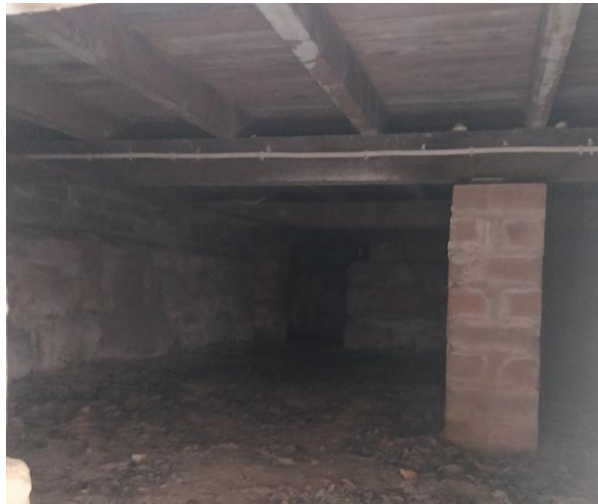
Figure 6. Crawl space under house with no floor insulation.
