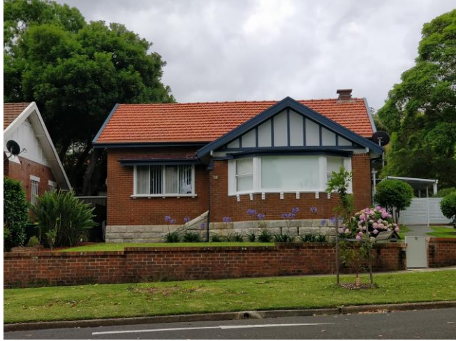
Figure 8. South side of the house with new installed aluminum windows on left and the original timber frame window on right.
