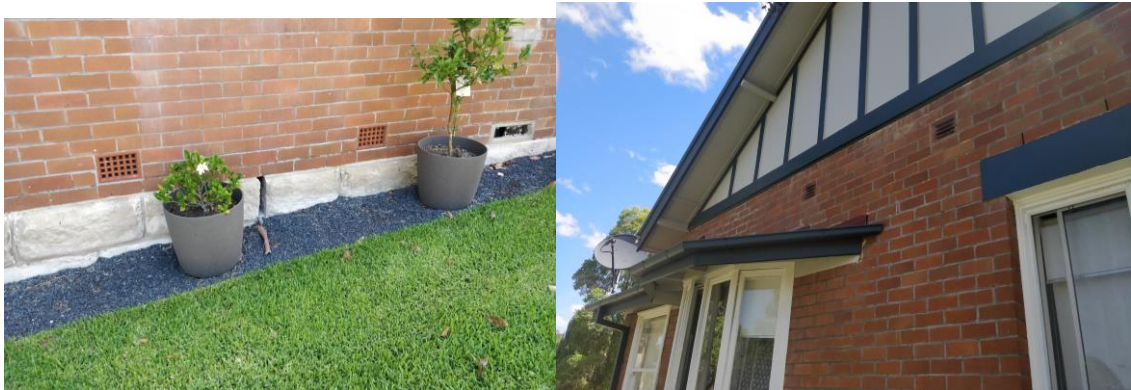
Figure 7. Natural air vents to allow the cavity air to circulate. Bottom of the wall to let air into the cavity (left), top of the internal wall (Right).
