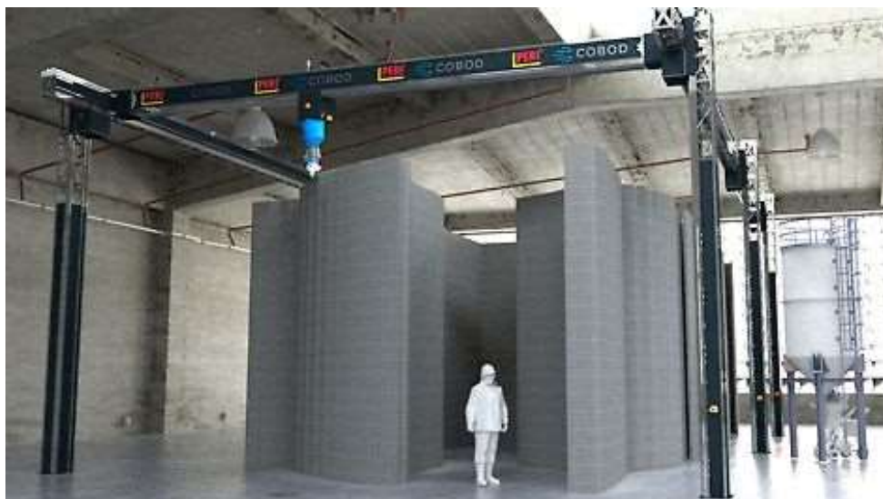
Figure 12. COBOD gantry 3D printer (Peri, n.d.)
