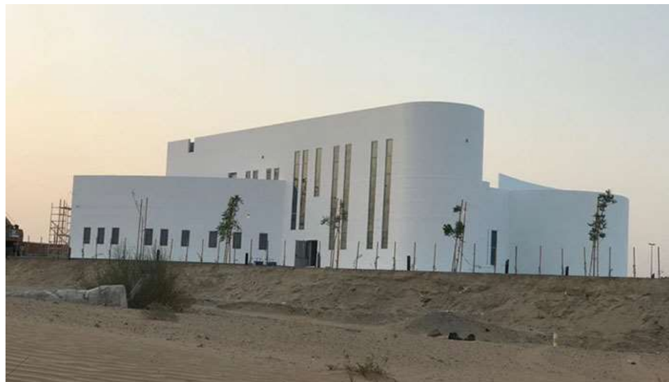
Figure 14. World's largest 3D printed building (Dubai, 2019)
