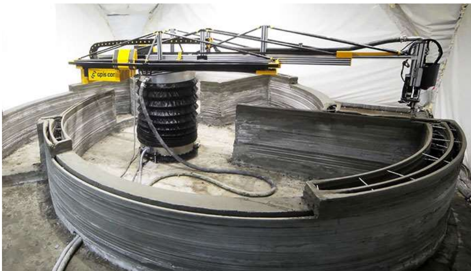
Figure 11. Construction 3D robotic arm printer Apis cor (Apis Cor, 2018)
