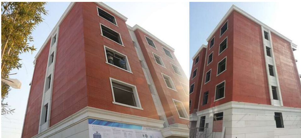
Figure 15. Five story 3D printed building (WinSun, 2015)
