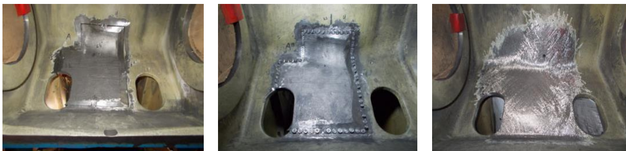
Figure 13. Pictures of a damage repaired by metal stitching
