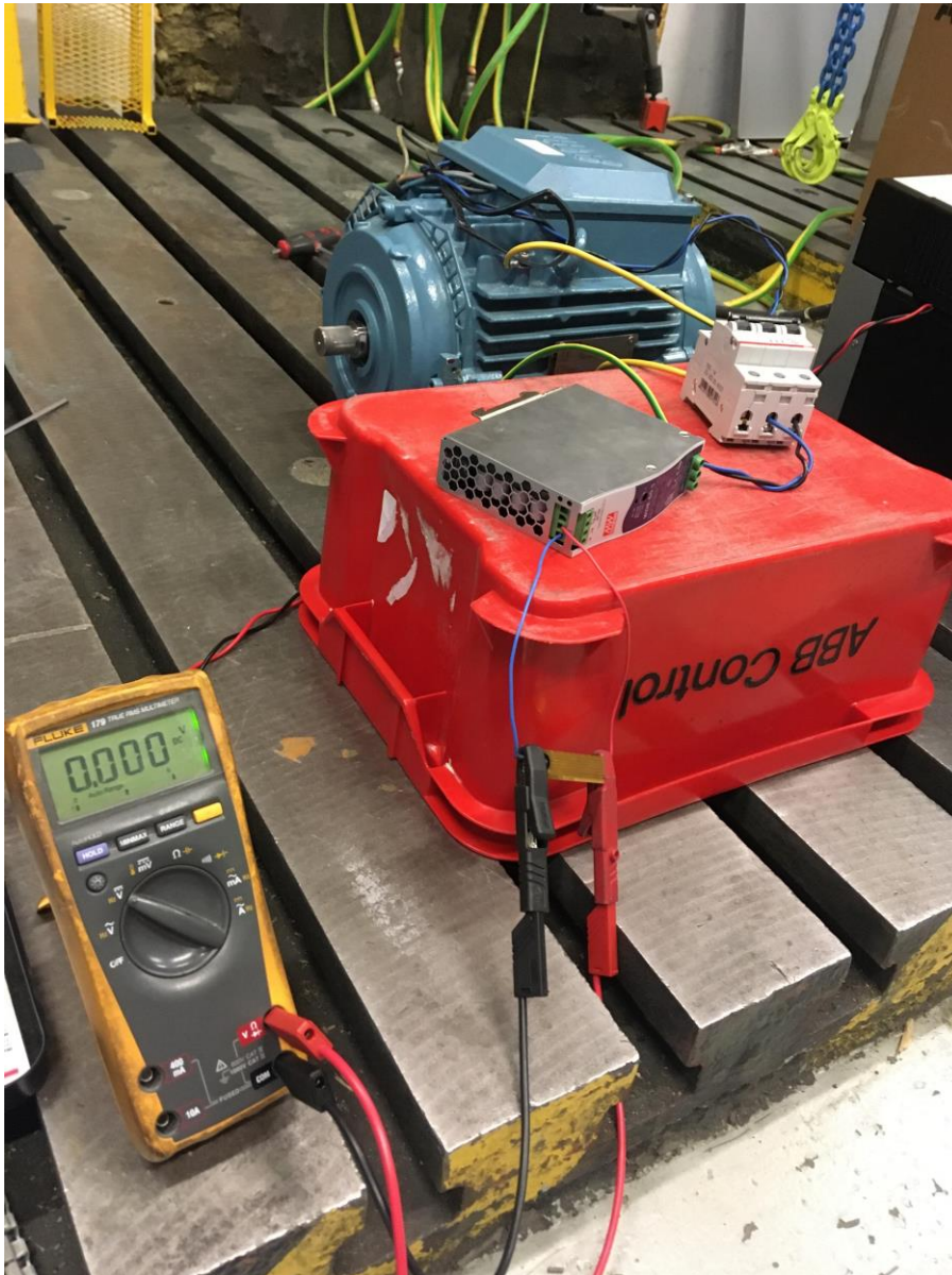
Figure 27. Connection of the power supply in the first test with a frequency converter.
