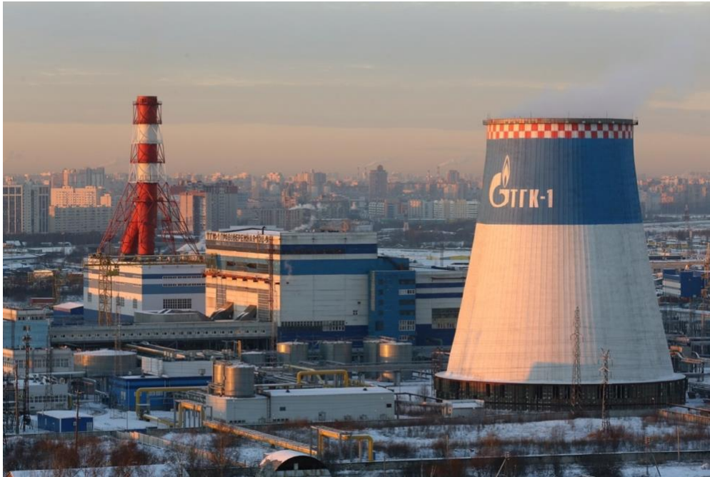
Figure 11. Cooling tower of “TGC-1” company. (Belayeva 2020.)
