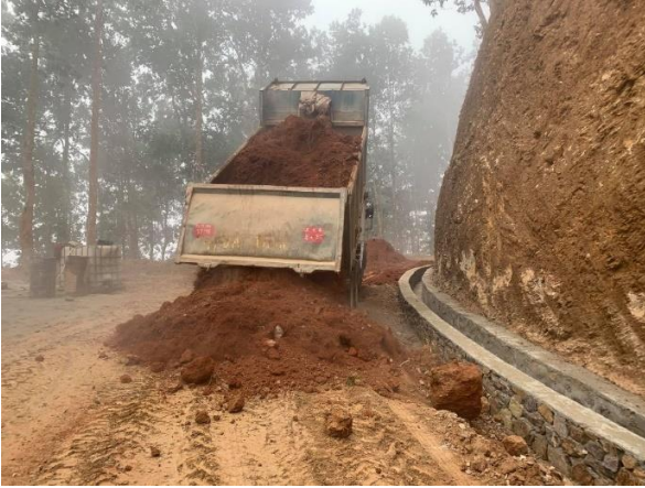
Figure 4. Image showing the tipper/truck unloading the soil of capacity 7.5m 3 .
