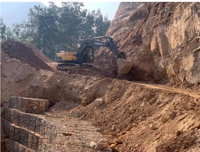
Figure 2. Excavation of rocks and soils from the road construction
