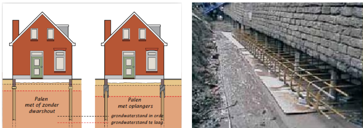
Figure 19 Left: buildings on wooden piles before and after pile head lowering; right: reinforcement of underpinning concrete structure ready to be cast (Photo: CJ Smith) (van Etten et al., 2007; VROM, n.d.)
