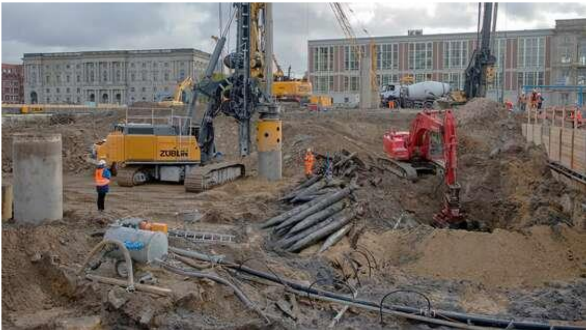
Figure 28 Removal of historical wooden piles in the Berliner Schloss site (Loy, 2012)
