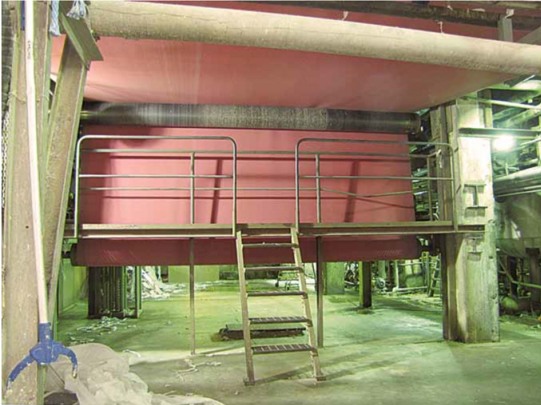
Figure 19 Picture of the working platform on which the accident happened. (Tapaturmava-kuutuskeskus 2012)
