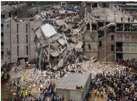
FIGURE 19: Rana Plaza following the collapse
