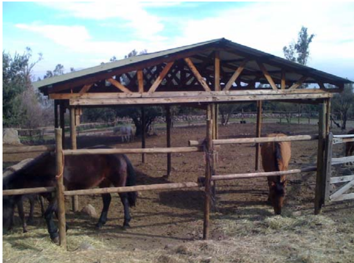
Figure 12: Wooden shelter to protect from the sun. Because it does not have any walls it does not protect from wind but in that area there is not so much wind it would bother the horses (Jokinen 2012)
