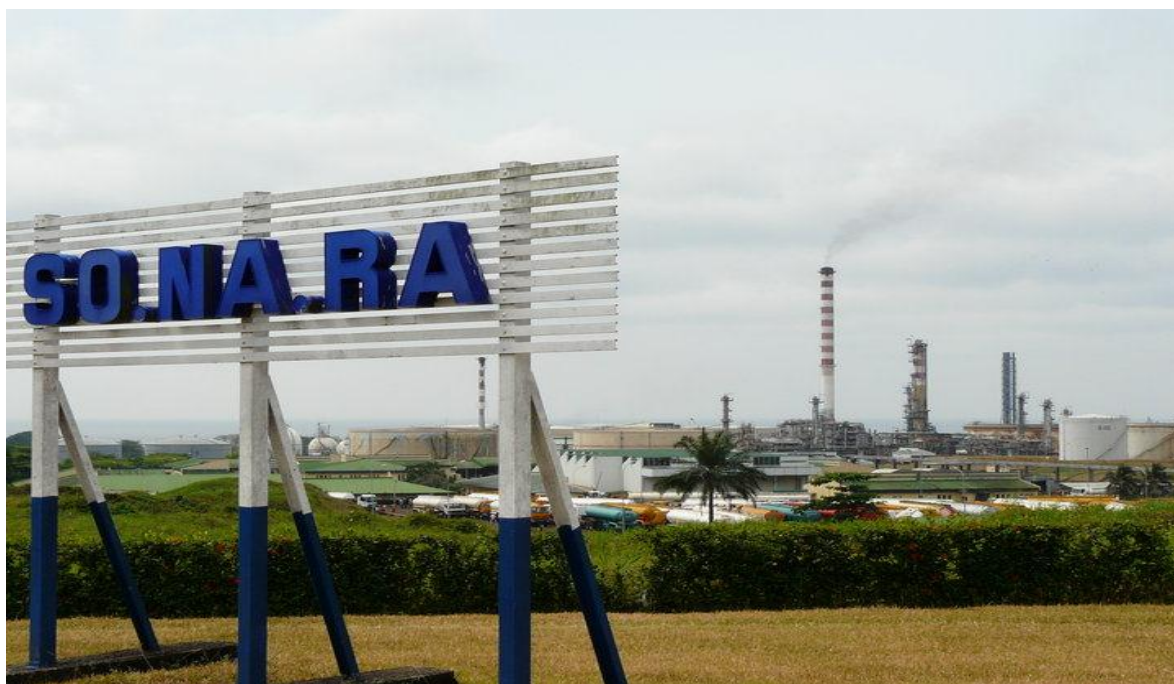
Figure 1: View of SO.NA.RA refinery.
