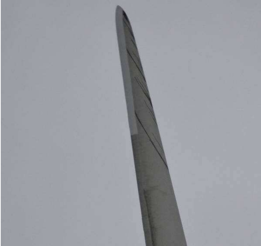
Picture 1. Newly coated area clearly visible. Note heavy blade pollution.
