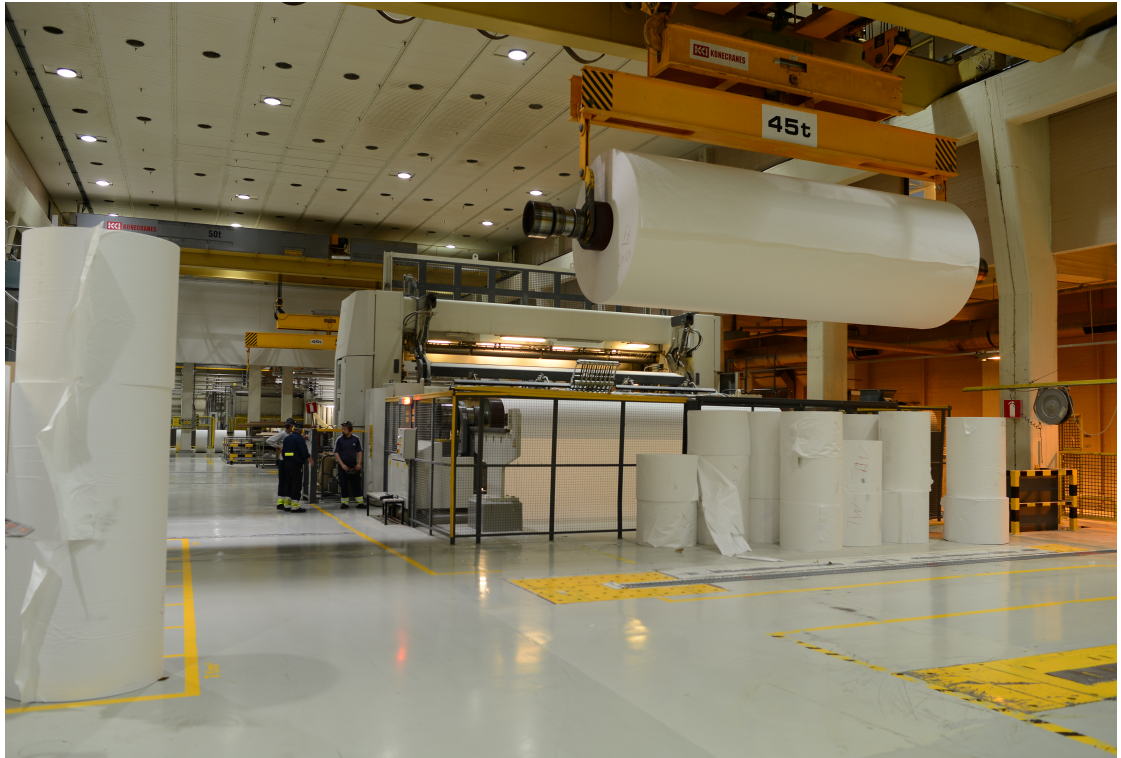
FIGURE 1. Paper machine reel being lifted to cutter
