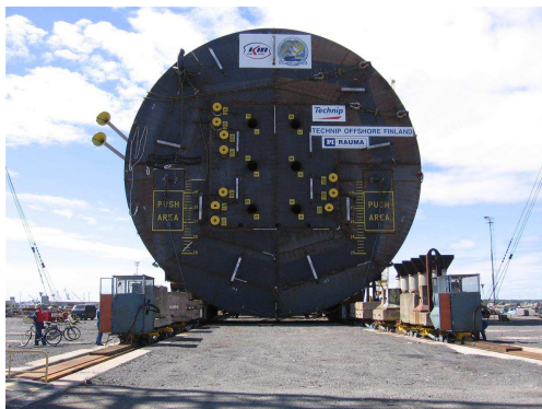
Figure 2.2.5: Push-pull units on the rails
