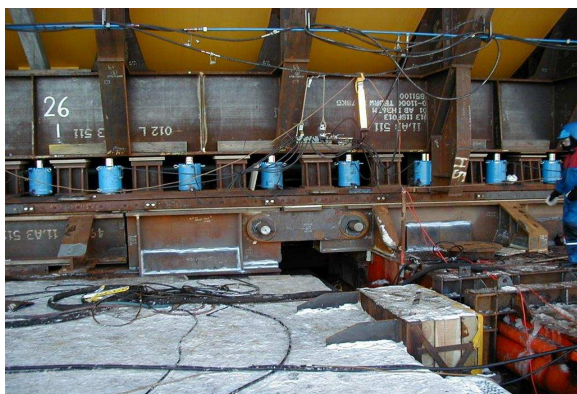
Figure 2.1.1: Skidding with hydraulics
