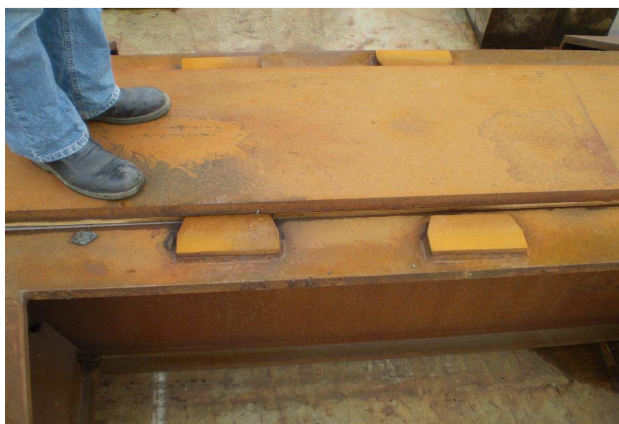
Figure 2.1.11: Roller plate on the skidding rail
