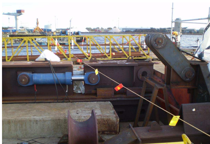
Figure 2.1.7: Connecting the link beam
