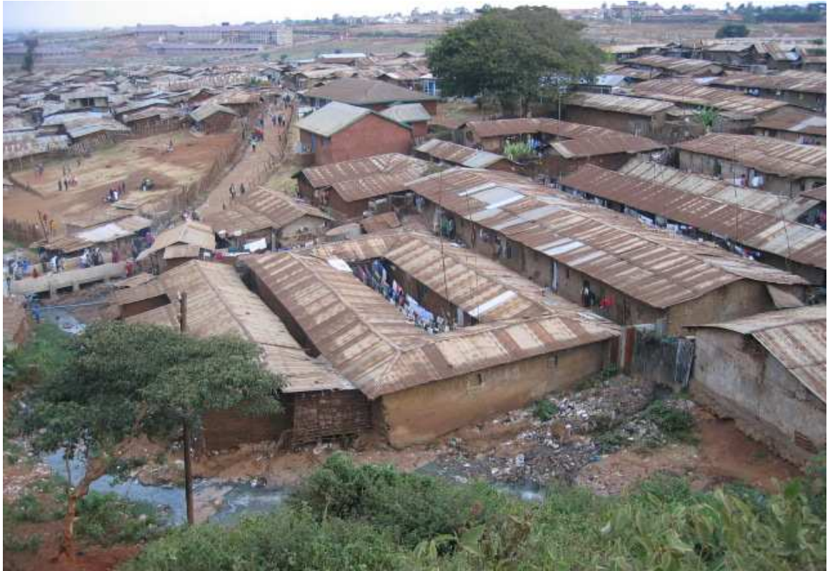
Picture 1: A section of Kibera slums with a raw sewage passing near the houses
