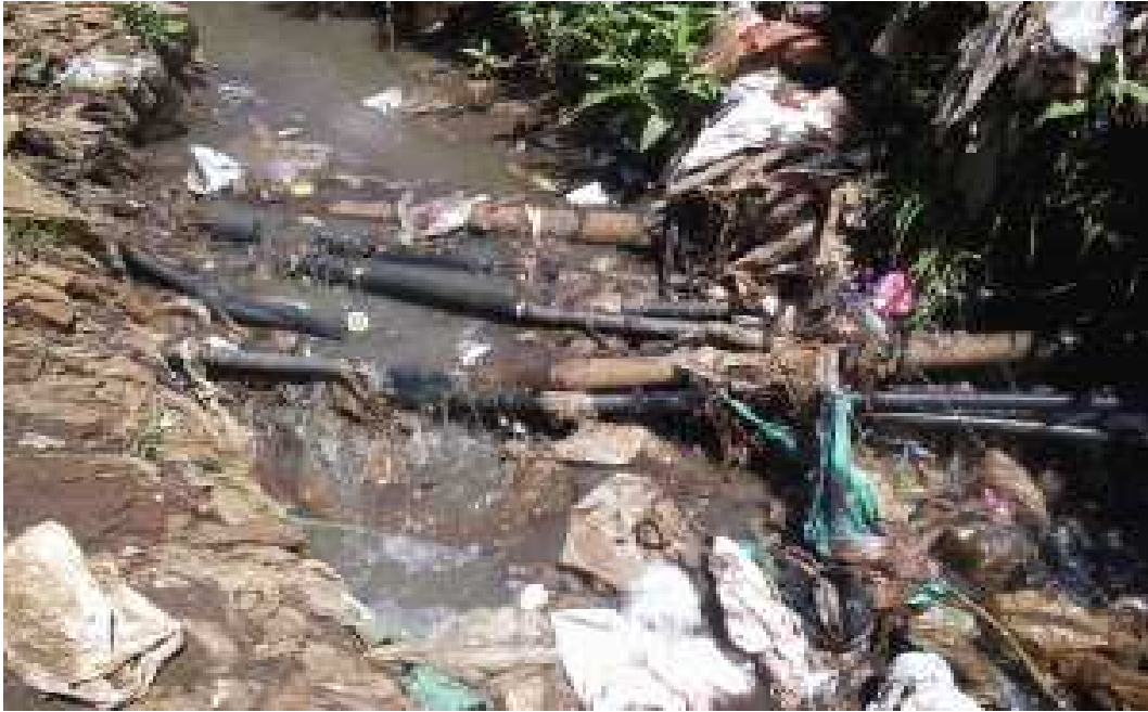
Picture 6: Sewage and water pipes flow together a suitable habitat for water-borne diseases.
