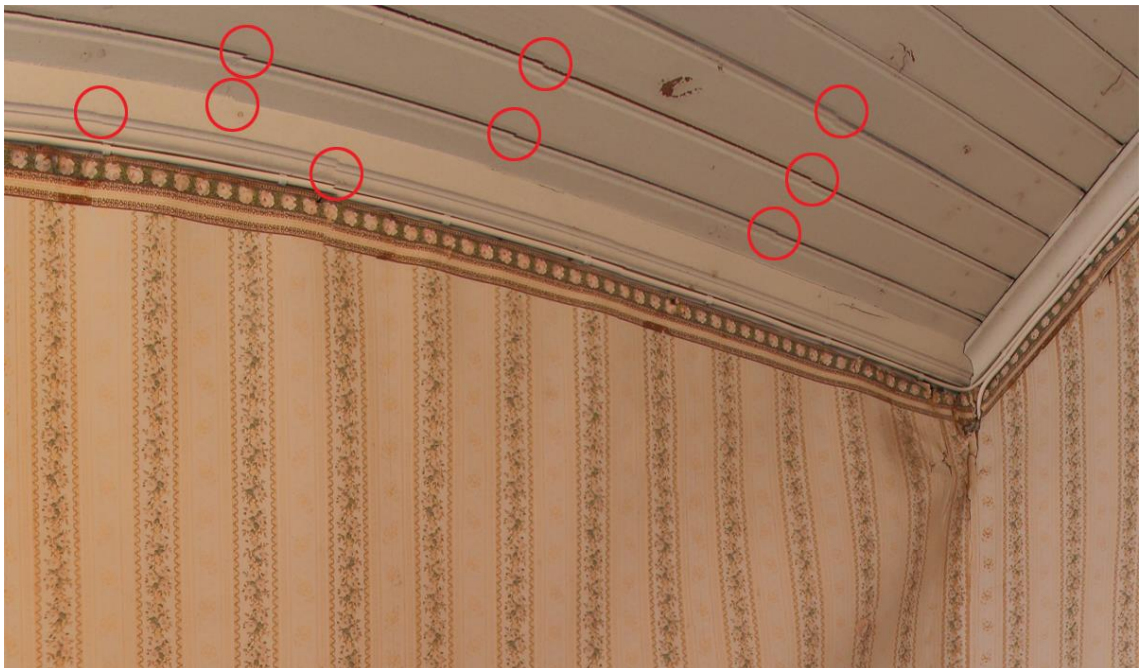
Figure 12. Image stitching errors around repeating patterns
