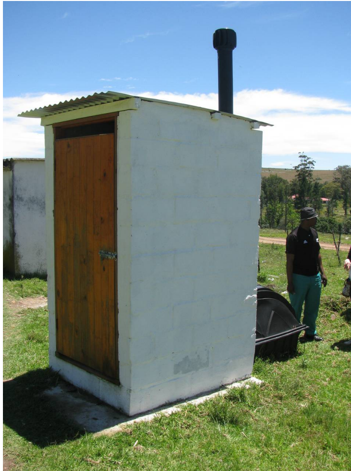
Figure 4: Composting dry toilet at Colingham farm, Makana, South Africa (Photo by Sofie Lundin).
