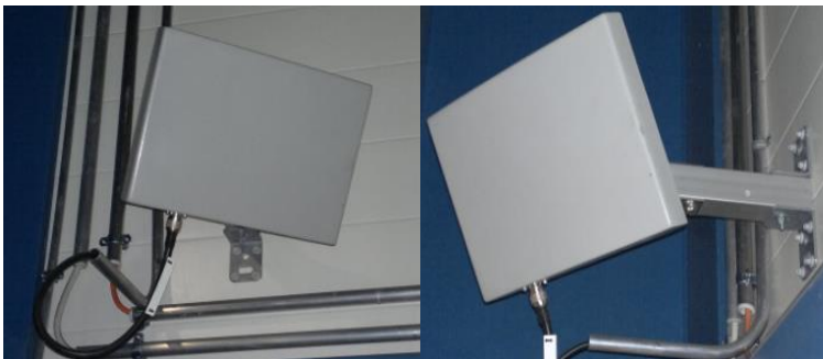
FIGURE 4. Aerial AV2100-CP antenna installation at F3 melt shop.
