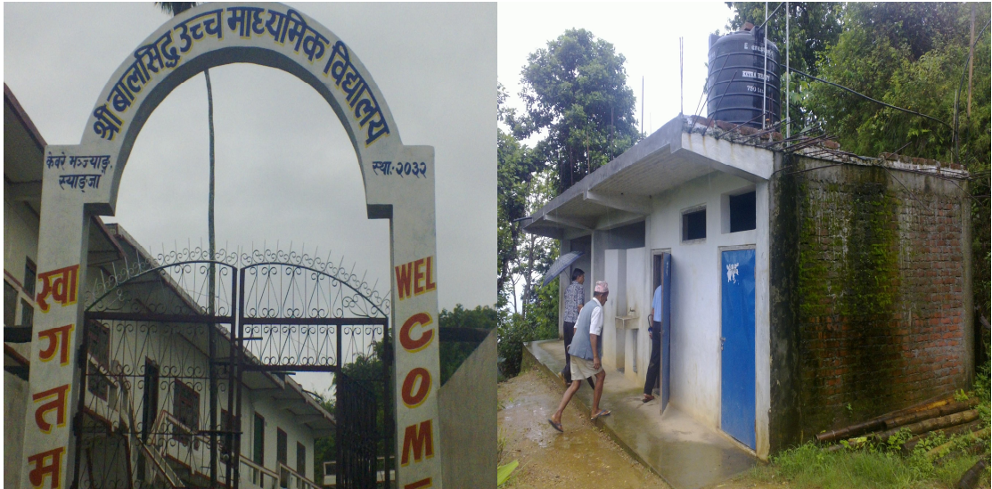
Photo 6: View of School Building and Toilet
