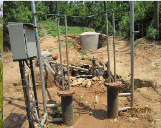
Photo 2: 2 nd pumping station, backfilling &
