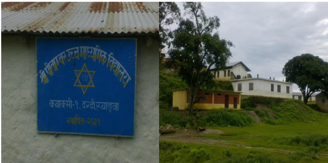
Photo 7: View of School Building and Toilet
