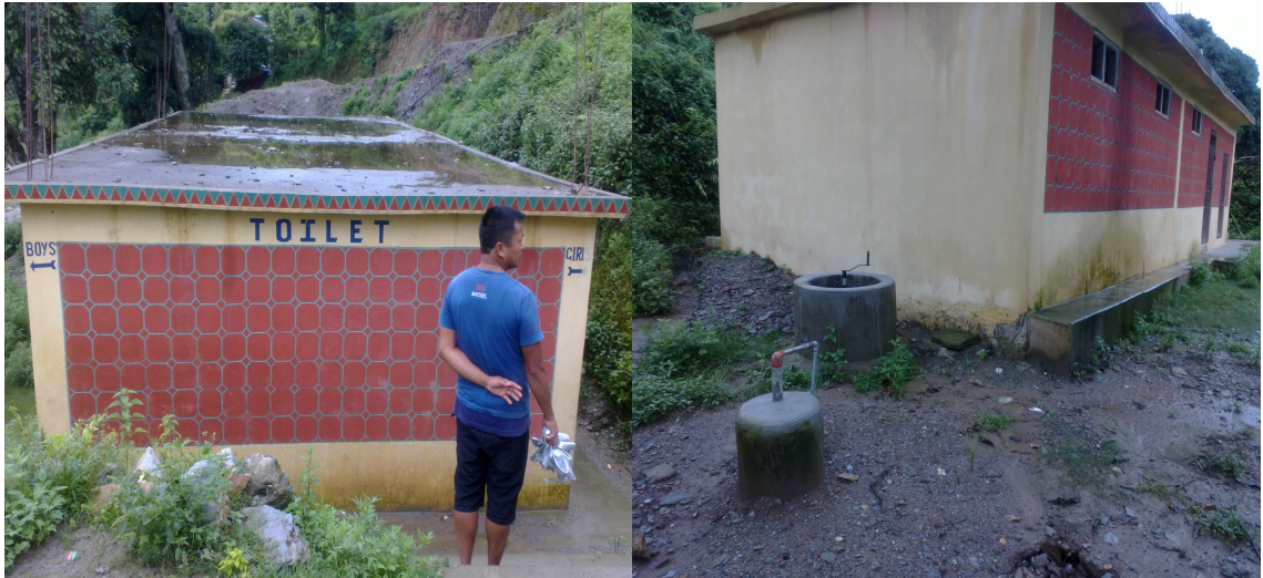
Photo 8: Institutional Toilet (at School) connected with Bio-Gas Plant (8 cum size)
