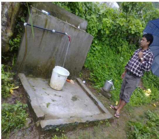
Photo 3:- Tap constructed by a HH as per choice
