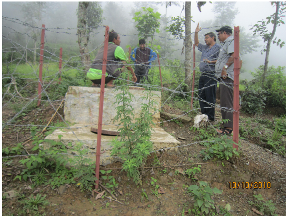
Photo 3: View of DC; Manhole cover properly fixed RVT; cleaning work needed
