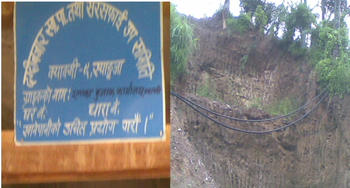
Photo 5:- Household ID No. (Blue Plate) provided to each HH Photo 6: Pipe exposed and hang ing at distribution line due to land
