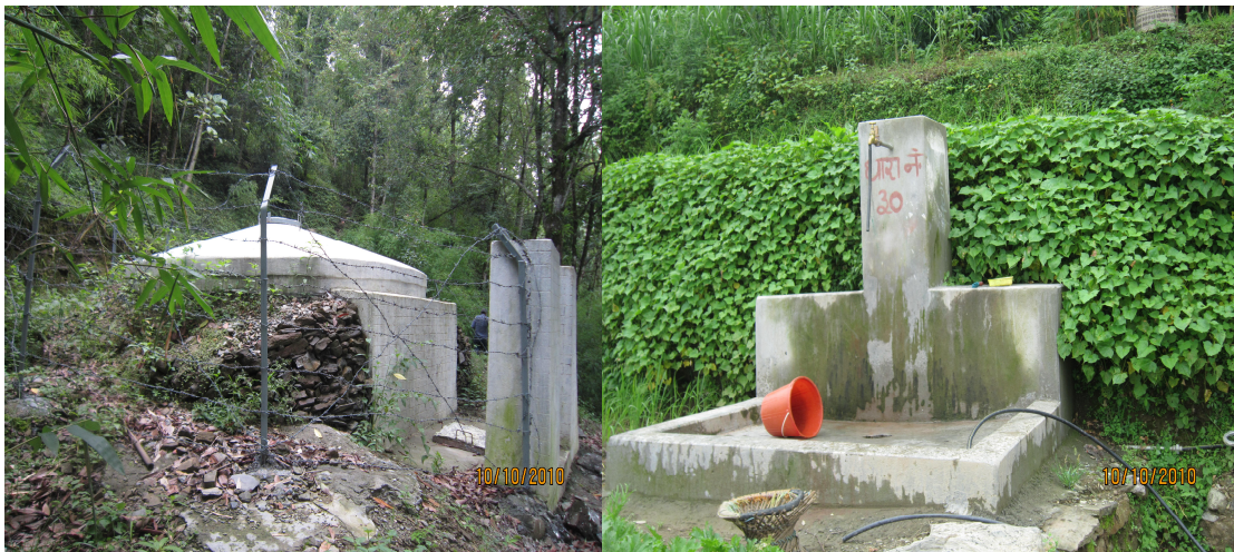
Photo 3: 2 nd RVT; good construction quality and fencing View of a functional Tap Stand
