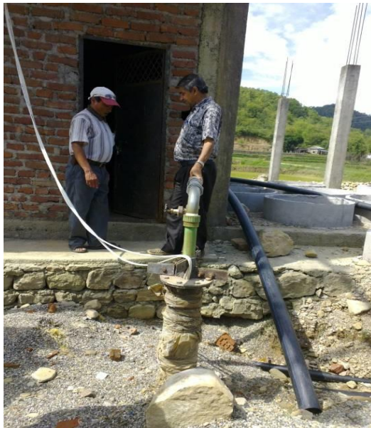
Photo 1: View of Boring site and pump House scheme
