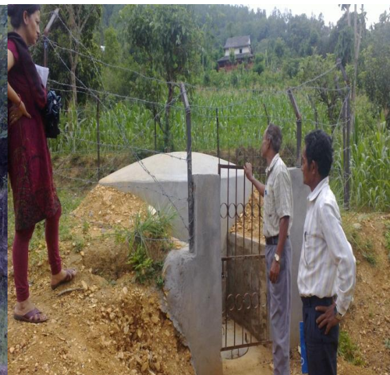
Photo 4: RVT with proper fencing.
