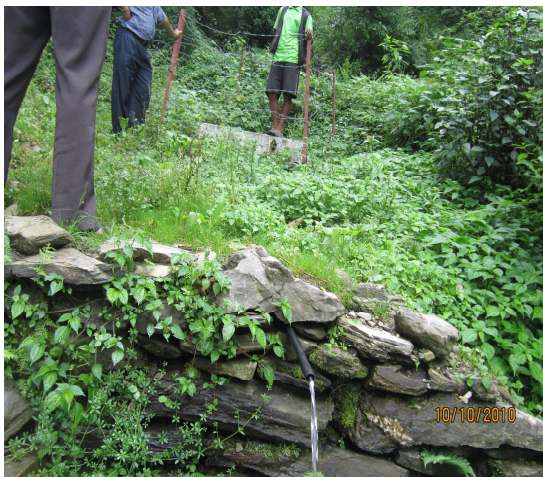
Photo 1: View of 1 st Intake and catchment Area Boulder packing at 2 nd Intake
