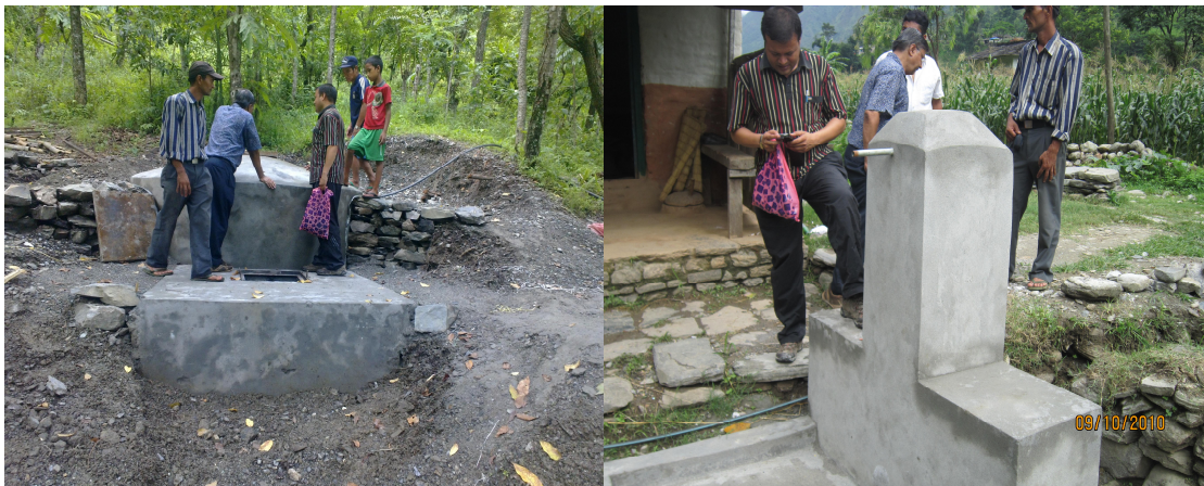
Photo 3: View of RVT, Fencing to be completed connection to be provided
