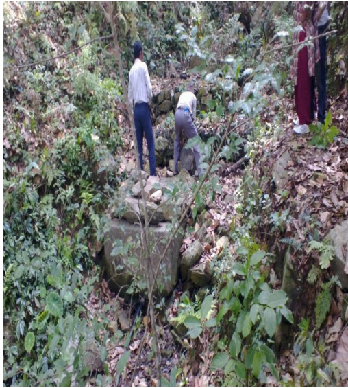
Photo 1: View of Intake/catchment; fencing needed pipe to be replaced
