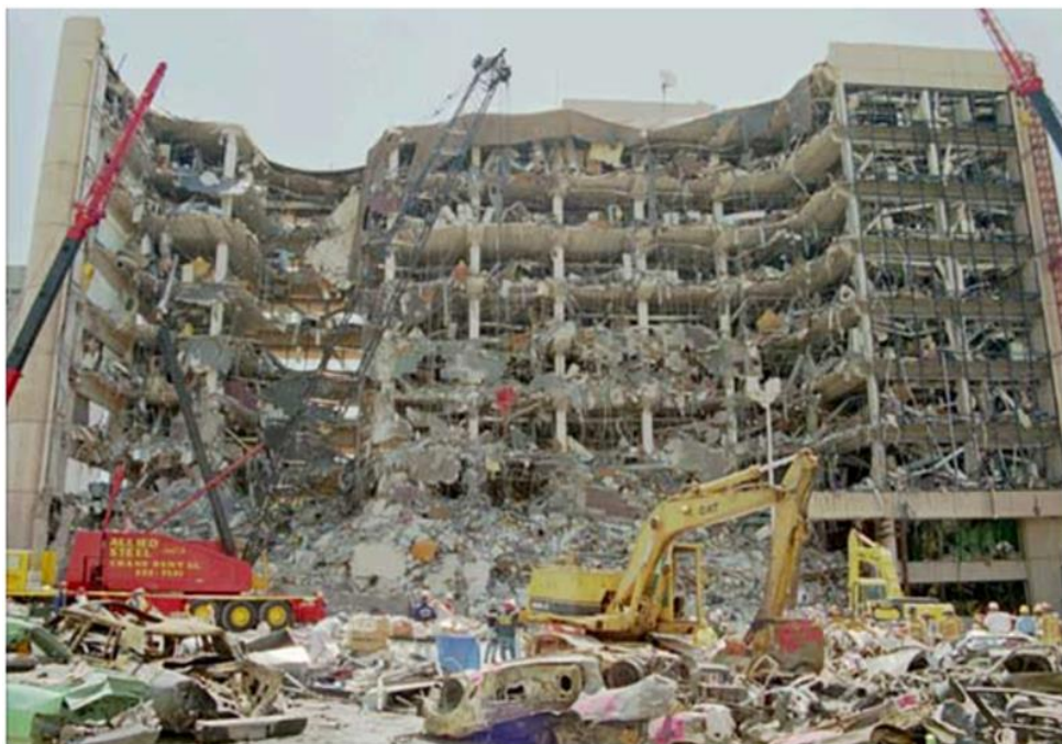
Figure 11. Murrah Federal Building after bomb attack
