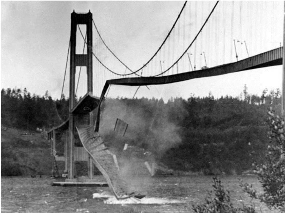
Figure 8. Tacoma Narrows Bridge after collapse
