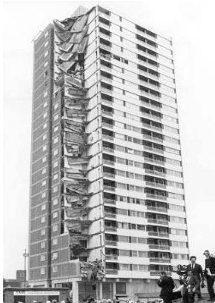
Figure 1. Failure of “Ronan Point”
