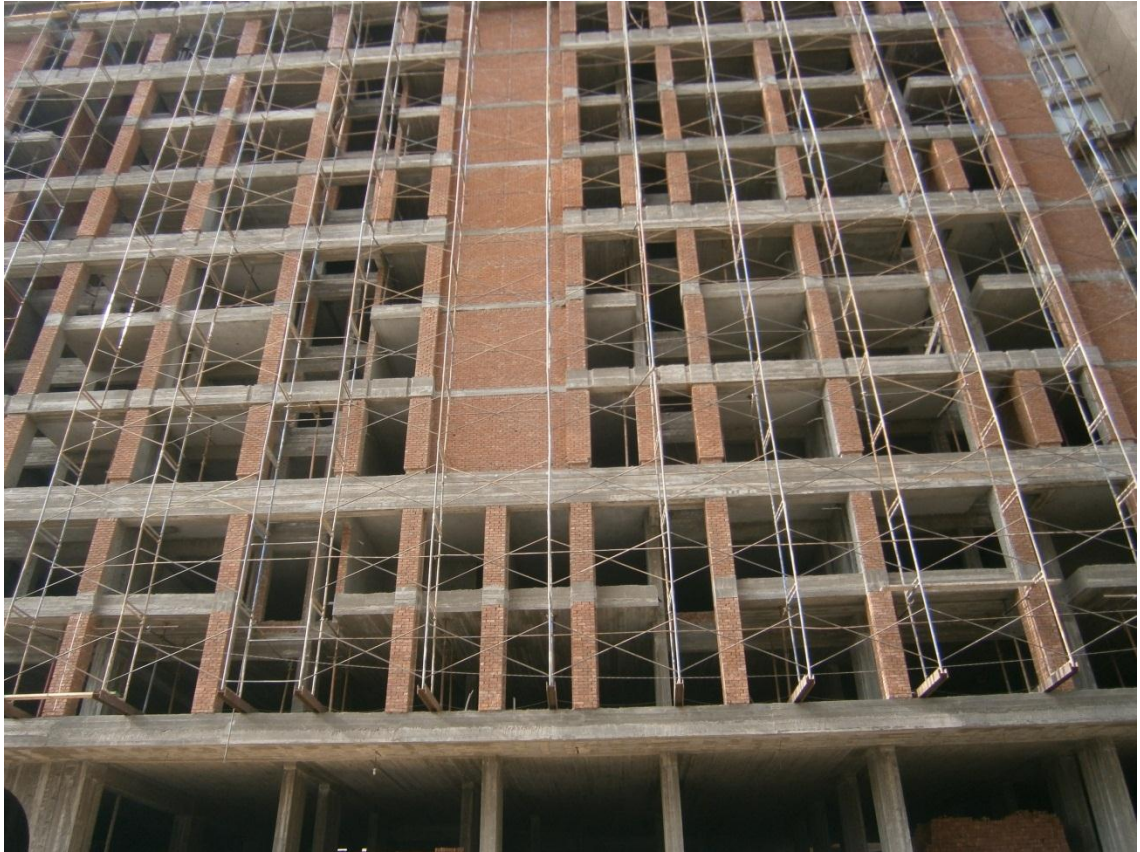
GRAPH 7. Metal scaffolding has been introduced lately to Egypt's constructors (Source: Author)
