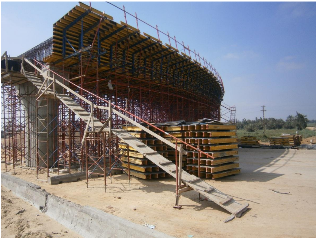
GRAPH 17. Steel tubes are rarely used for bridges scaffolding, will that last forever? (Source: Author)
