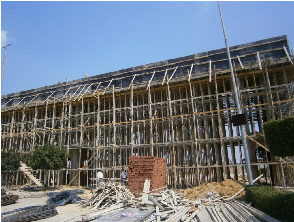
GRAPH 16. Bridge construction in the midway between Alexandria and Cairo. 6 meters long fillery is used intensively (Source: Author)
