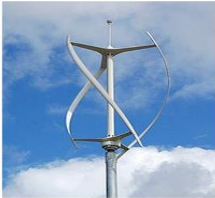
Figure 2. Vertical axis wind turbine (Bracken Meyers 2013)
