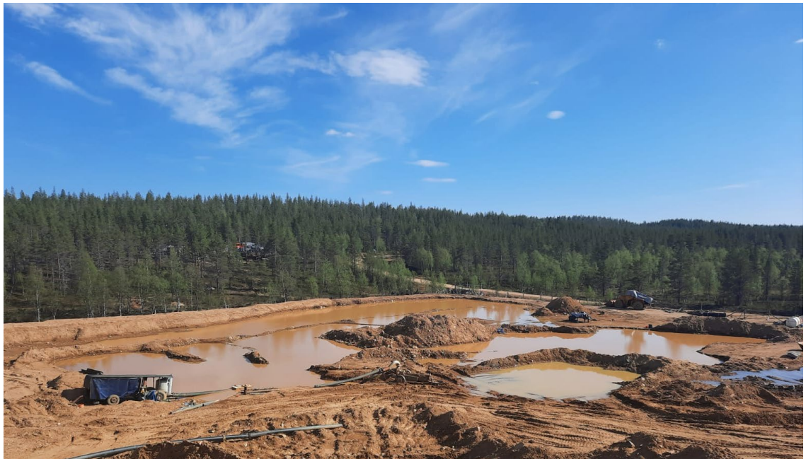
Figure 4: Settling ponds after 10 months, claim "Jokela". (Photo: E. Takaluoma 2021)
