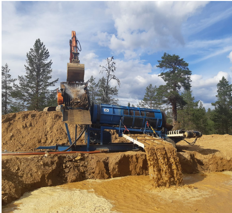
Figure 2: Gold processing unit at claim "Selperi" (Photo: E. Takaluoma 2020).
