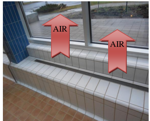
FIGURES 19-20. Supply heated air from grids in the pool's space
