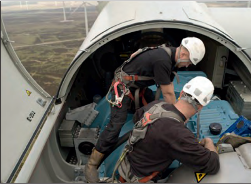
Figure 4.5. Complicated maintenance work, high in the nacelle. (Siemens Press Pictures 2010)
