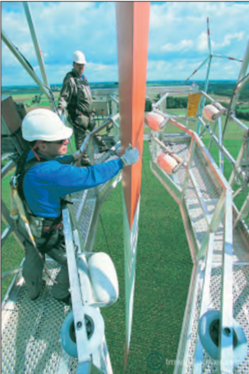
Figure 4.6. Maintenance team inspecting a rotor blade with the help of a lift (Courtesy of LM Wind Power, lmwind-power.com s.a.).
