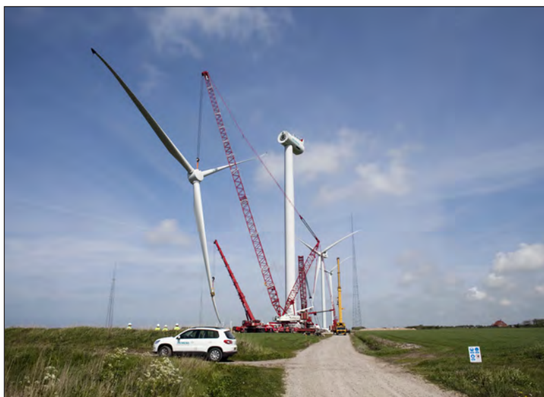
Figure 4.3. Demanding lifting operations with special equipment (Siemens Press Picture 2009)
