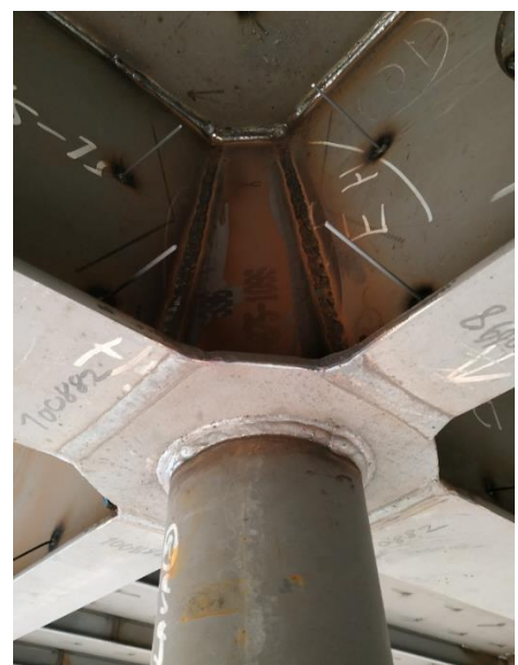
Figure 46. The pillar to the deck beam's webs connection in production.
