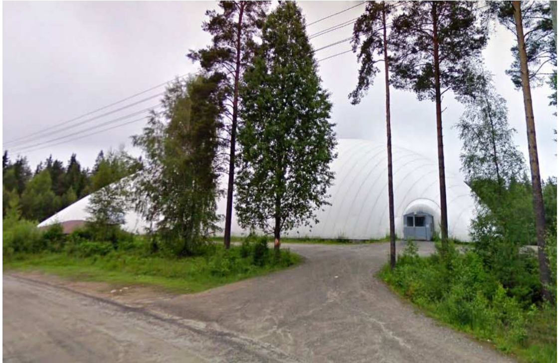
FIGURE 7. Air-supported structure in Mikkeli, Finland
