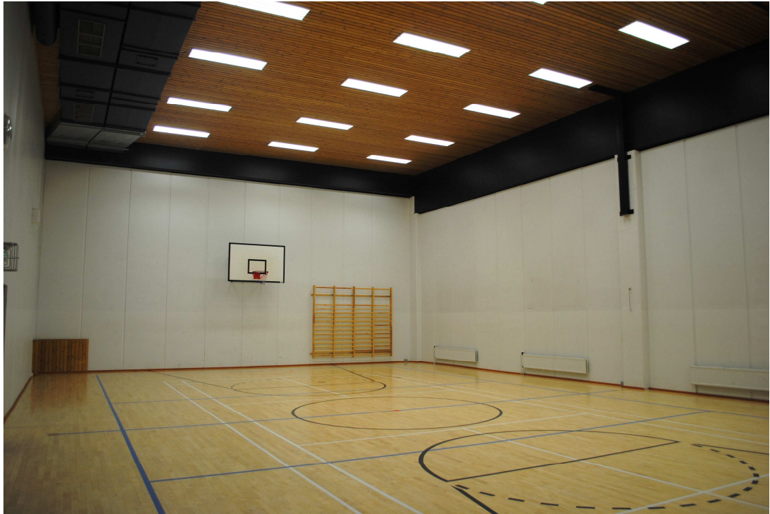
FIGURE 10. General appearance of sport hall in D-building of MUAS
