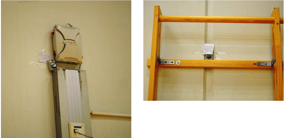
FIGURE 24. Mounting of data loggers on the walls
