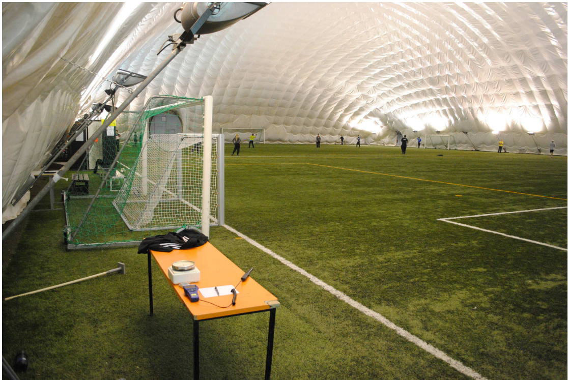
FIGURE 23. Monitoring of indoor climate in air supported structure
